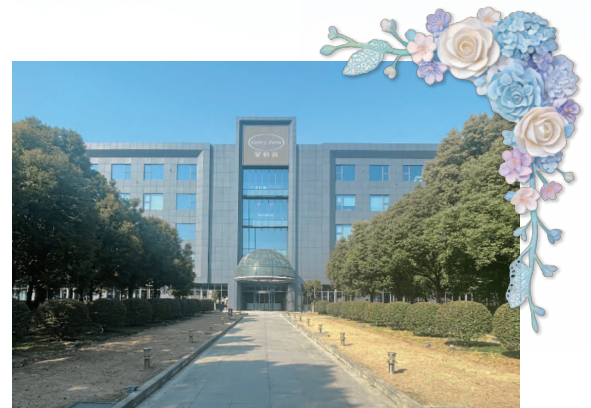
Changzhou Industrial Park
